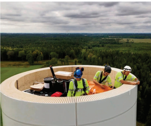
Engineers work on the construction of the world's tallest wooden turbine tower
