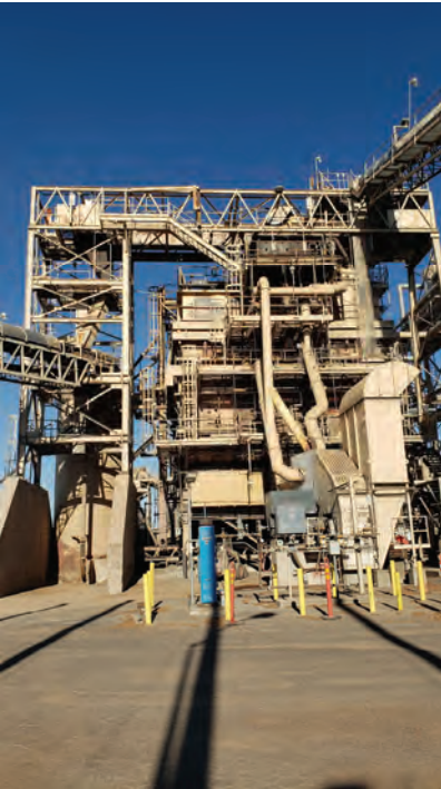
Wood biomass plant.
